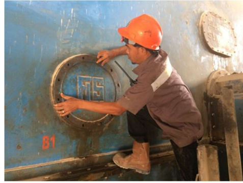
Gambar 4. Proses membuka cover bearing
